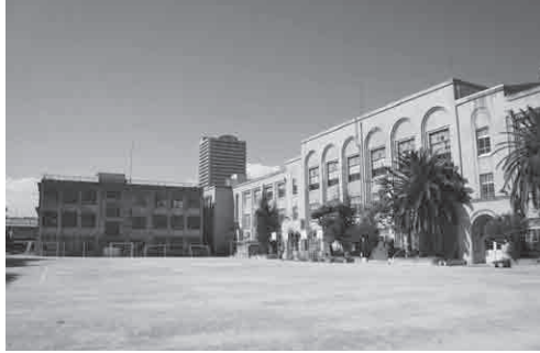
FIGURE 5 School buildings after the quake (courtesy of the Futaba Center)
